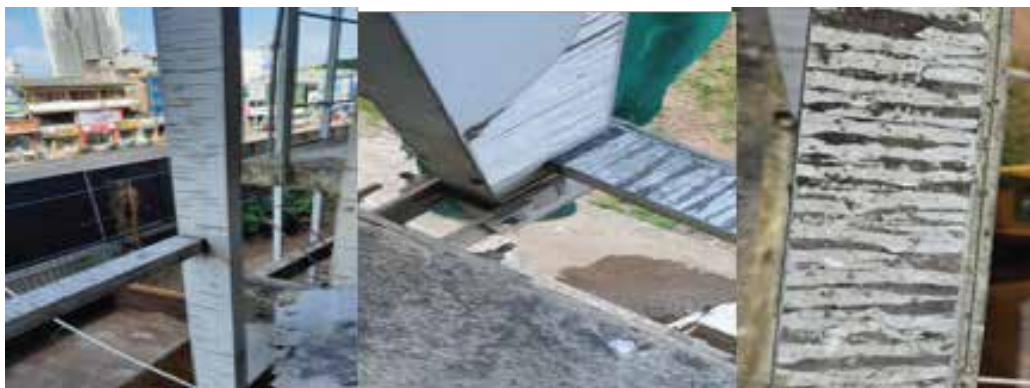
Image 17: leaving the protective tape on the fabricated profile for a longer period than required
