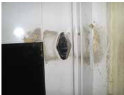
Image 18: Pasting unapproved tapes
