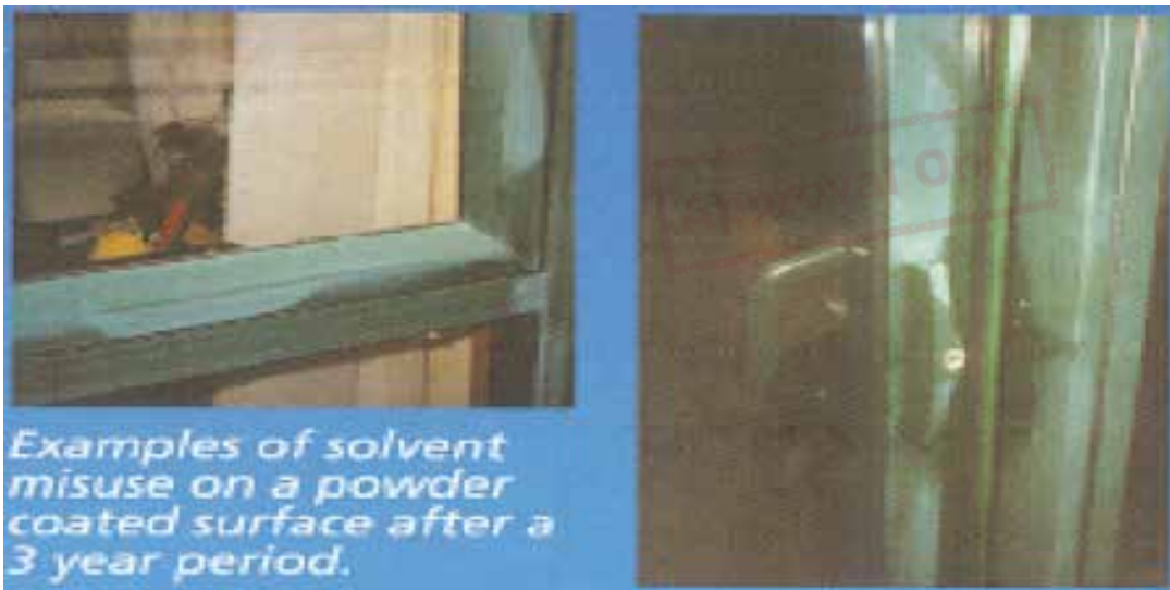
Image 22: Solvent misuse on powder coated surface after 3-year Period
