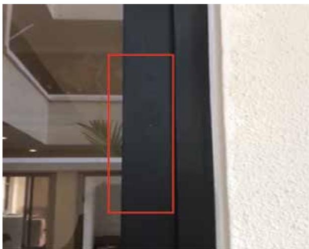
Image 10: Printed content on the protective tape transferred onto the profile surface
