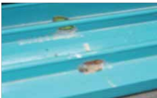
Image 14: Proper cleaning of weep frame holes
