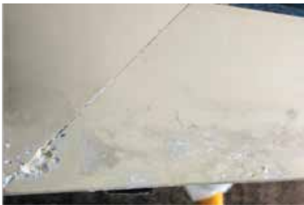
Image 16: Bimetallic/ Galvanic Reaction
